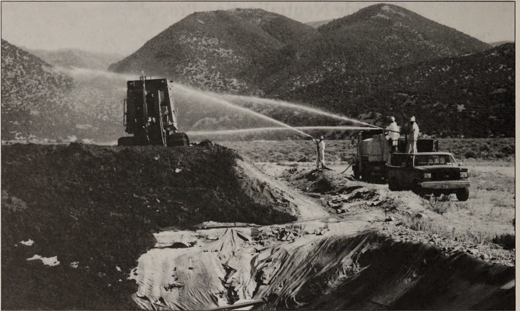
Figure 5. The trailer-mounted hydromulcher behind the pickup was used to apply reagents, with the additional water needed to reach the desired concentration being sprayed on by the BLM fire pumpers. Note the protective clothing being worn
